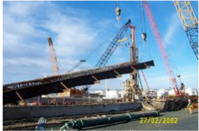
Using a "strong back" for raising cage
