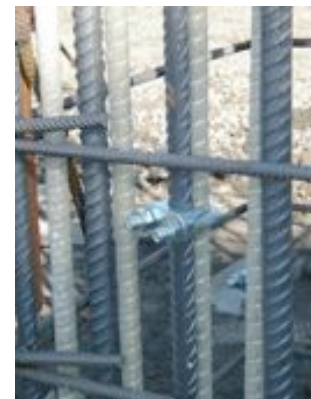
Clamp to connect steel to FRP bar for lifting
