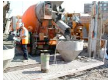
Tremie Pipe filling D-Wall
