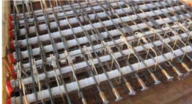
Fig. 2: The segmental precast deck elements included post-tensioning ducts, steel reinforcing bars, and GFRP stirrups. The GFRP bars were detailed to extend above the finished deck
