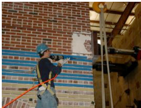
Structural tuck pointing of masonry
