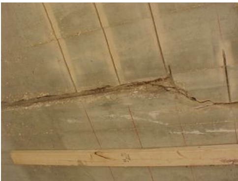
Structural crack stitching of crack in bridge deck
